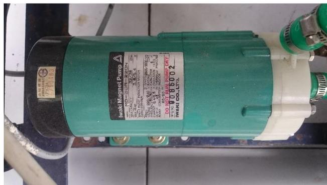
**Gambar : 3.6** Pompa Iwaki Mangnet Pump MD-30R-220N
