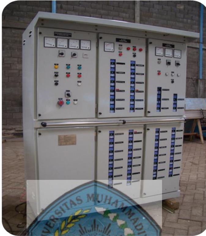
Gambar II.10 : *Emergency SwitchBoard*
