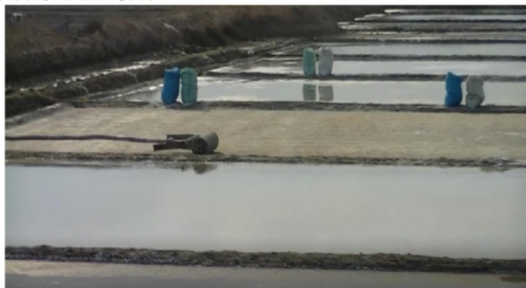
Figure 2. The soil compaction process using the selender
